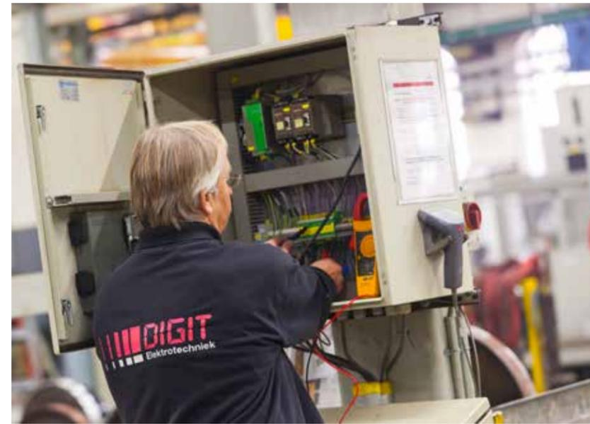
Measurements in a switch case
